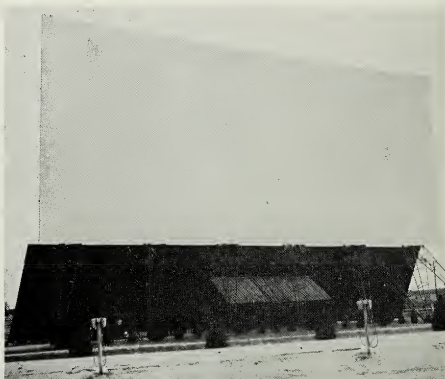
steel construction and is 120 feet wide and 52 feet high. It has five coats of paint to insure even light distribution and clear, sharp picture images.
